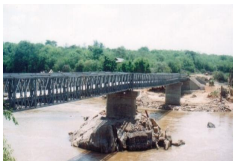
The Bailey bridge
