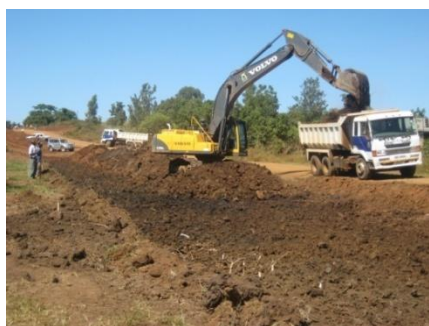
Top soil stripping to spoil
