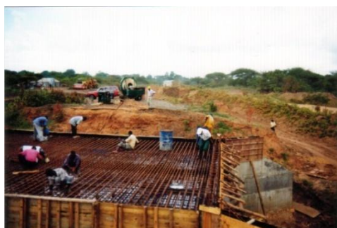
Reinforcement to top slab box culvert
