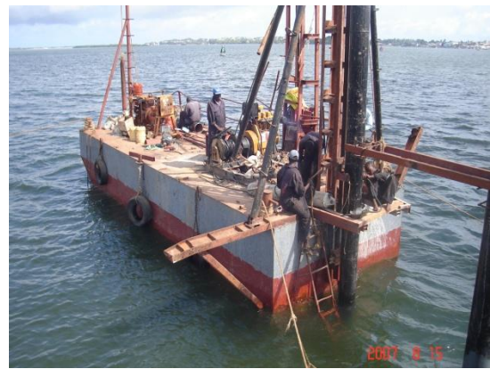
Piling barge in sea
