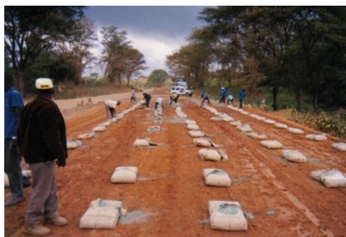
Cement stabilizing of approach road
