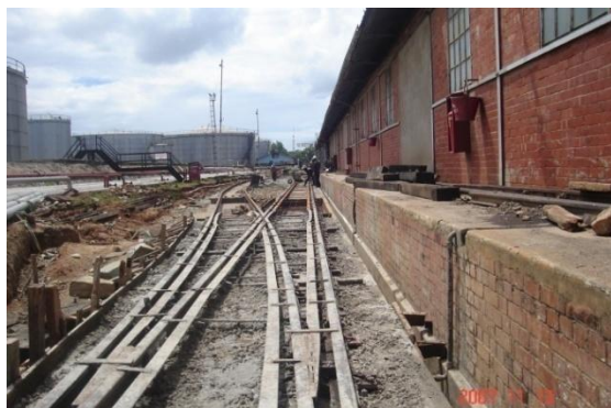
Turnout track laid on base concrete
