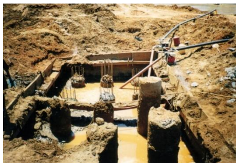
Head treatment to bored piles
