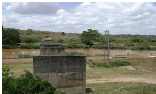
Complete Piers South end
