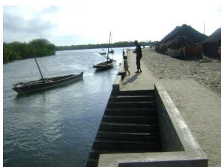
Seawall stair case
