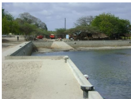
Completed section of seawall
