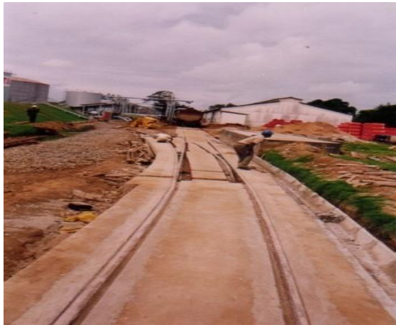
Rafted Track turnout laid in concrete
