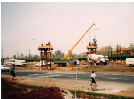
Working under traffic
