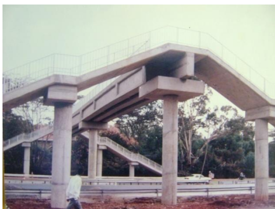
The completed structure
