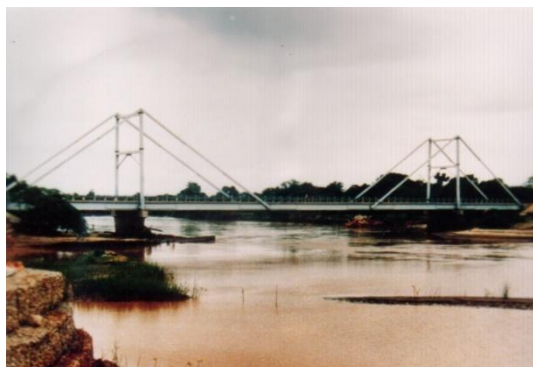
The bridge with protection on left
