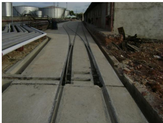
Turnout track cast in topping concrete
