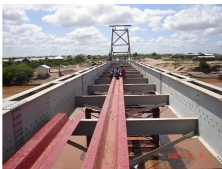
Cross beam and troughing installation
