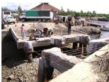
Breaking of jetty for reconstruction
