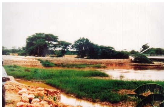
Bank protection in gabions
