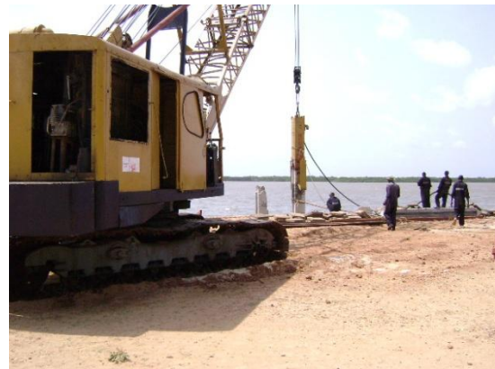
crawler crane with diesel piling hammer
