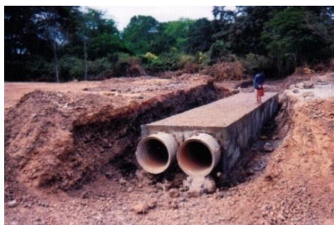
Twin cell 1200mm pipe culvert
