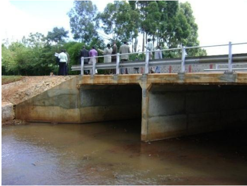
The 3 cell 5m x 2m box culvert
