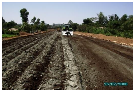
Base stabilization with cement
