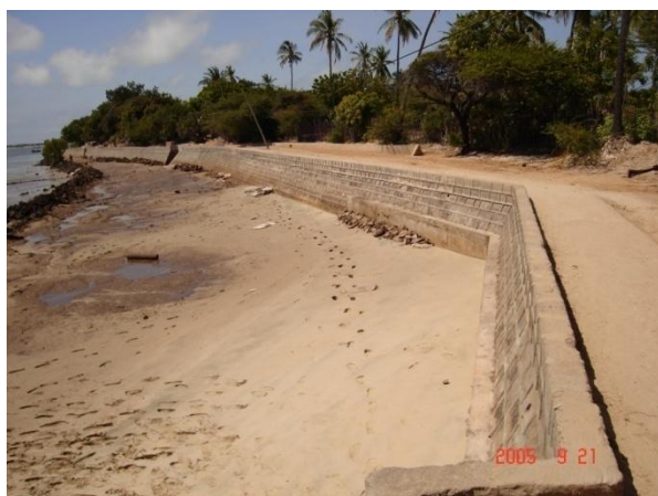
Completed seawall section concrete blocks
