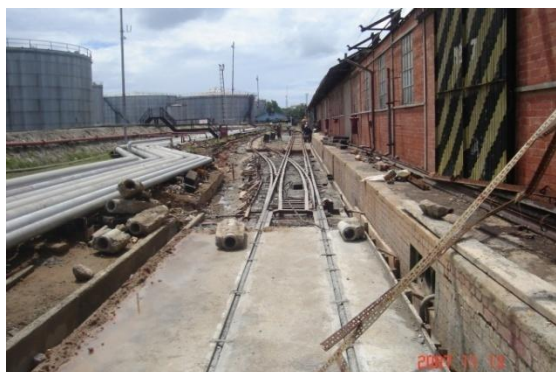
Plain track cast in topping concrete
