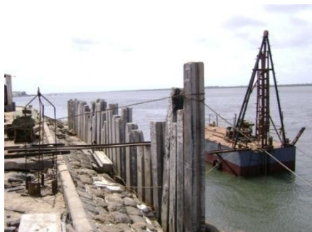
Driving concrete sheet piles
