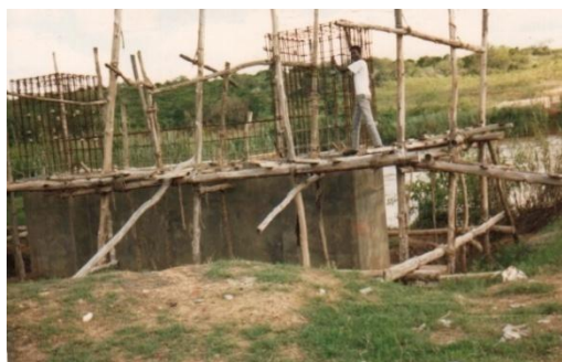
Concrete construction to pier
