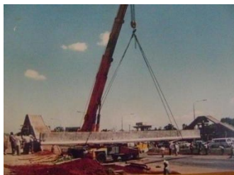
Hoisting of precast girders
