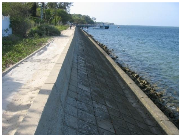
Completed sea wall section armour blocks
