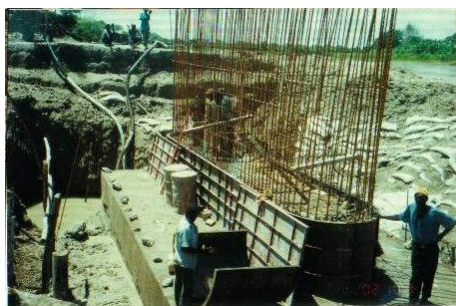
Concrete construction to pier base and stem
