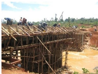
Scaffolding and form work to bridge
