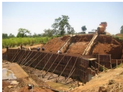
Scaffolding and form work to bridge
