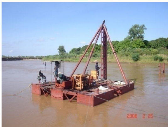
20 ton pontoon with piling equipment
