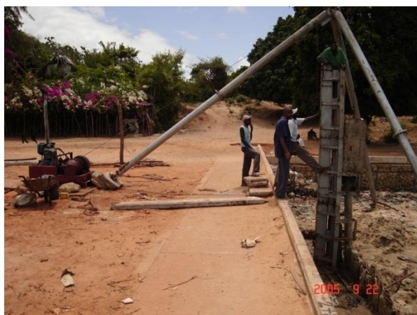
Driving Concrete sheet piles
