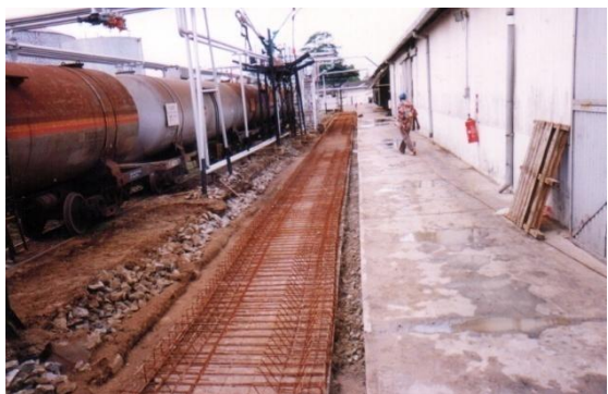
Steel reinforcement to base concrete
