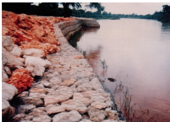
Bank protection and groynes
