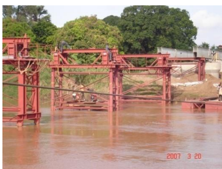
Temporary trestles to deck construction
