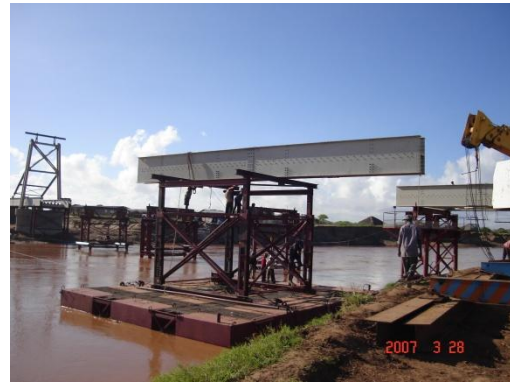
40 ton pontoon barge with lifting trestle
