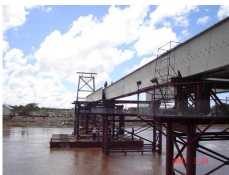
Stiffening girder installation
