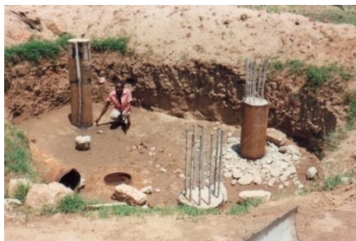
Concrete bored piles
