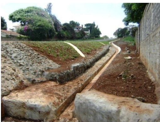
Drainage works and embankment
