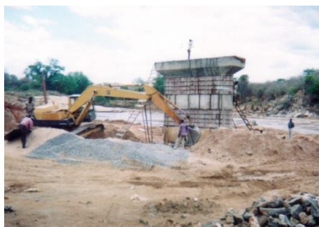
Concrete construction pier
