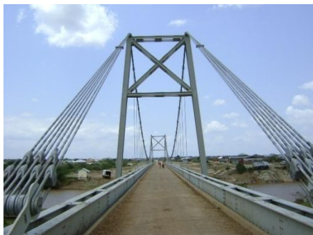
The completed bridge deck
