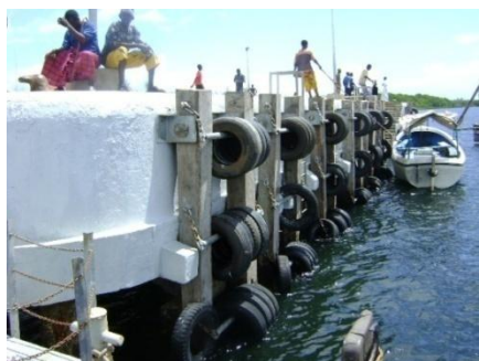
Rehabilitated jetty with fenders
