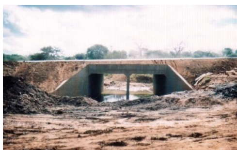
The completed 2 cell 4.5m x 4.5m BC
